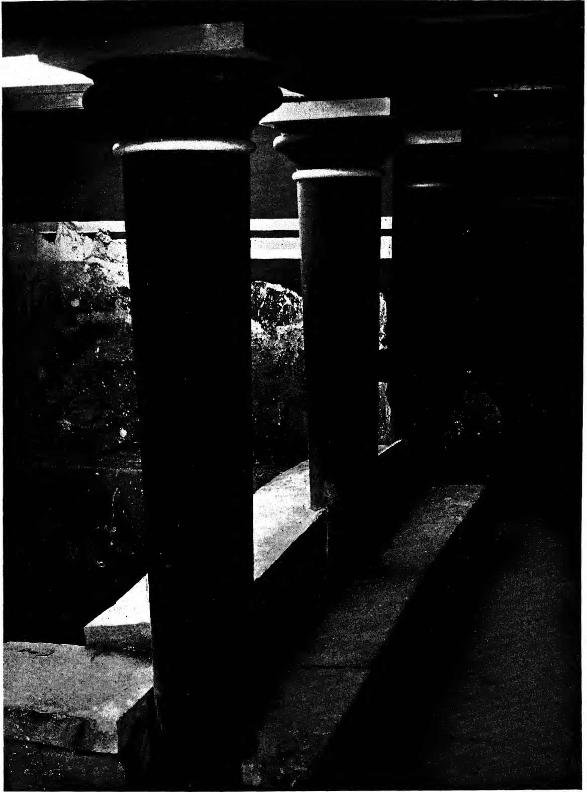
FIG. 883. VIEW OF 'LUSTRAL BASIN' WITH BALUSTRADE AND ADJOINING BENCH, THE CARBONIZED WOODEN COLUMNS RESTORED.
